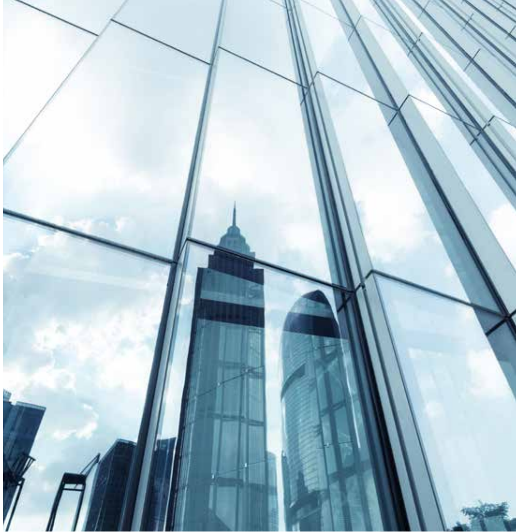
irregular facade elements requiring analysis
